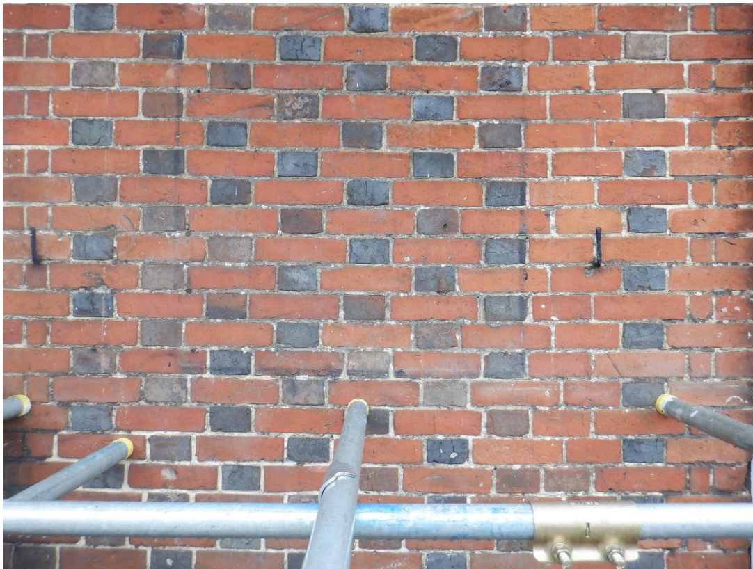
Plate 9. Street View 2023 brick detail mostly Flemish Bond with overfired headers
