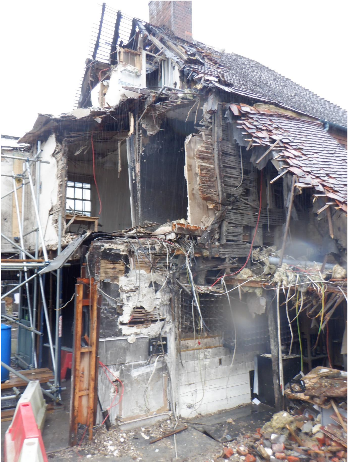
Plate 10. Interior (looking north)
