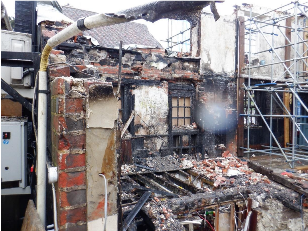
Plate 12. Interior (looking North)
